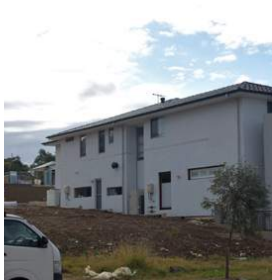
Figure 28: Building to the edge of lot, minimal setbacks, no space for shade trees. Photo: from the project image bank, collected by the research team during site visits.
