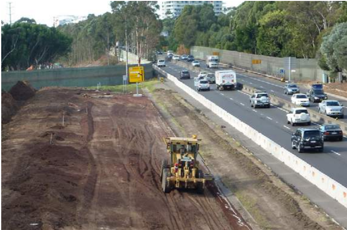
Figure 16: Privileging major roads – clearing the way for M4 widening at Strathfield involved the removal of urban forest planted after the building of the F4 in the early 1980s. Photo: Cathy Jones. Reproduced with permission. https://strathfieldheritage.org/2017/01/31/m4-motorway-history/
