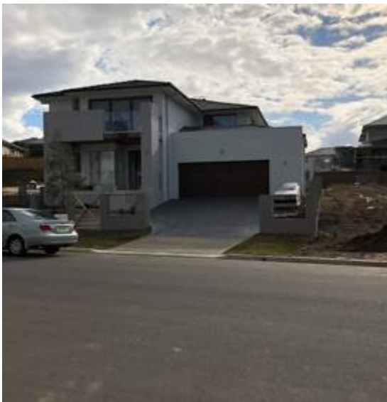
Figure 27: Impervious, unshaded dark surfaces, unshaded narrow balcony, spaces designed for car rather than pedestrian access. Photo: from the project image bank, collected by the research team during site visits.
