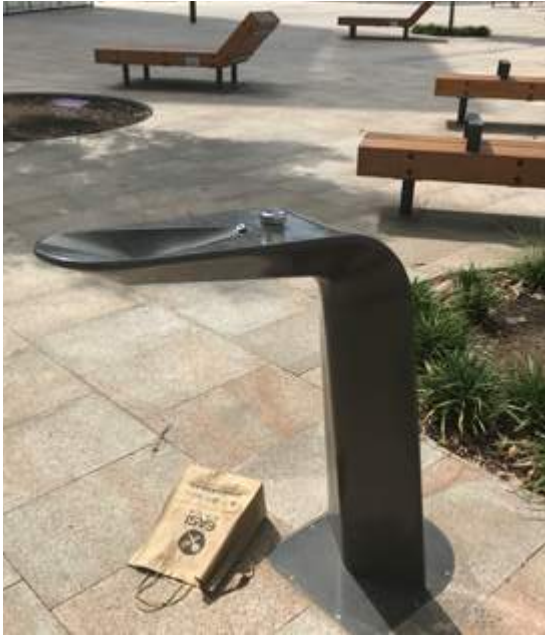
Figure 31: Unshaded water fountains get hot in the sun and are unpleasant to drink from. Photo: from the project image bank, collected by the research team during site visits.
