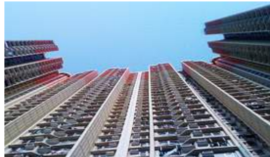
Split-system air conditioning units on the façade of a residential high-rise in Kowloon, Hong Kong. Source: https://www.tugraz.at/en/tu-graz/services/news-stories/tu-graz-news/singleview/article/architektonische-loesungen-statt-klimaanlagen/
