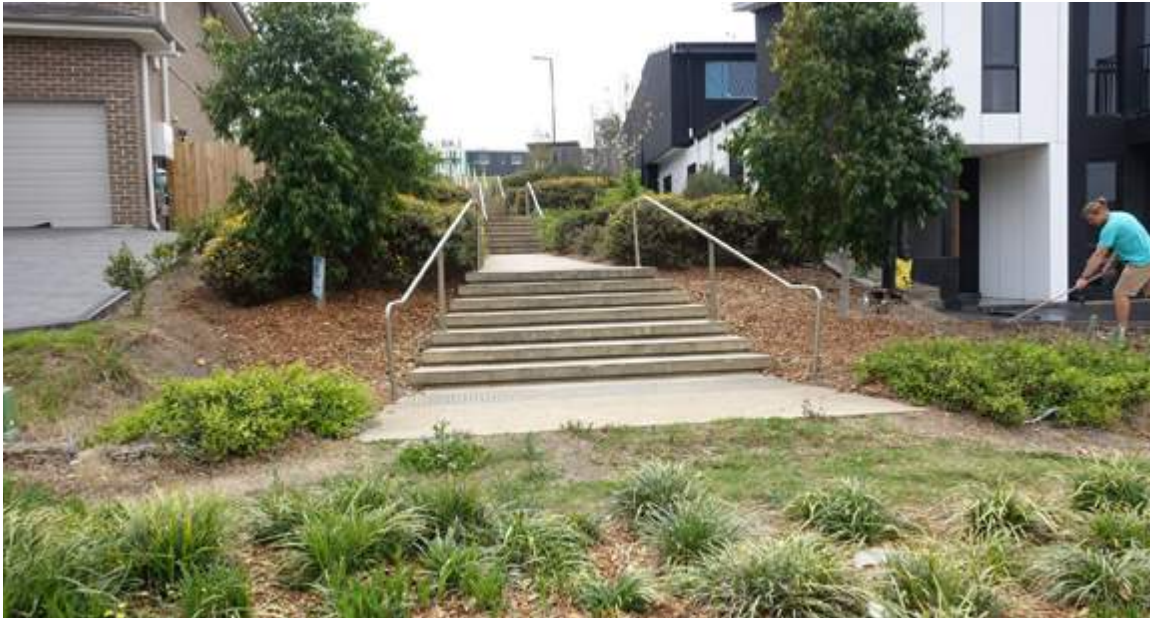
Figure 29: Lack of universal access; paths that do not connect to destinations. Photo: from the project image bank, collected by the research team during site visits.
