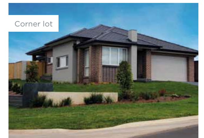
As both sides act as the 'front' of the home, the design and landscaping must emphasise and 'wrap around' the corner as well as look out onto both streets.
