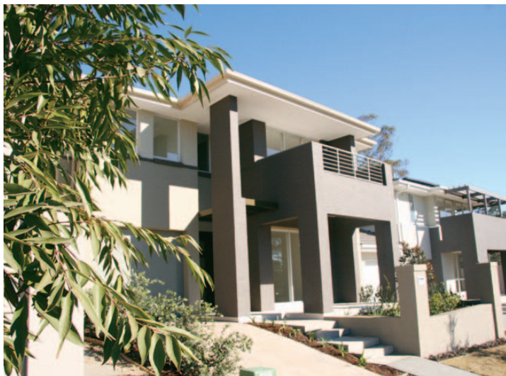
Layering and detail added to the front facade can add amenity as well as improving the appearance of the house from the street.
