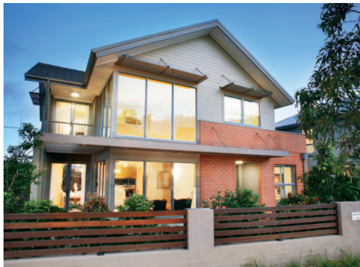
Simple geometric forms, shade structures and a well designed fence are combined here to create a quality home that sits comfortably in the street.
