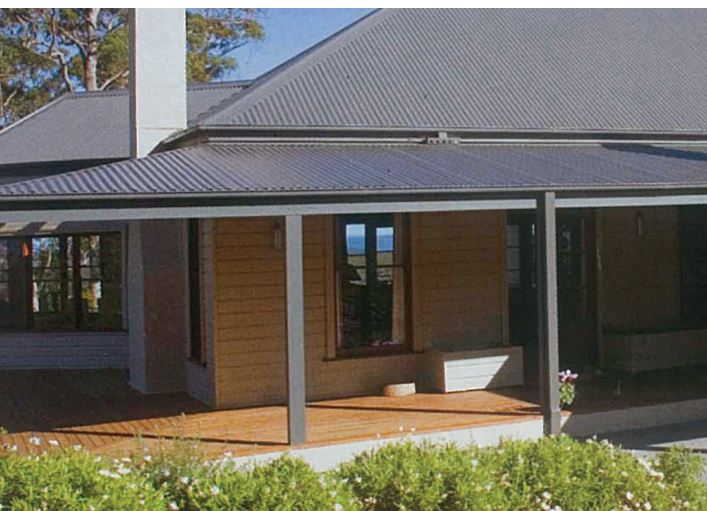
Generous verandahs provide additional living space as well as sheltering windows and doors from sun and rain.
