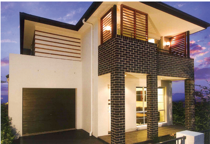
A single garage door makes significantly less impact on the front facade of the house than a double one. It also allows a narrower driveway and a larger area of soft landscaping.
