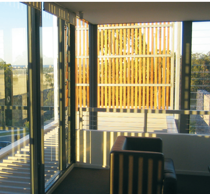
Well designed screens can add to the aesthetic appeal of the home as well as improving privacy.
