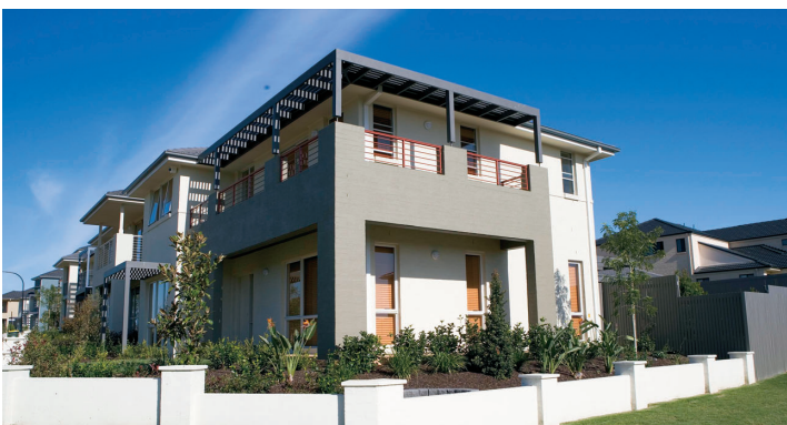
A wrap around balcony and garden enables this corner house to address both streets.
