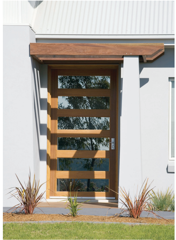
Quality features added to an otherwise simple house can improve its aesthetic value for a reasonable cost.
