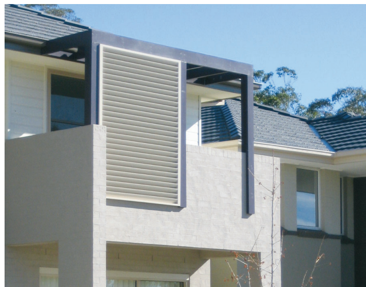
Side facades, especially, may benefit from screens to provide privacy between neighbours while still allowing larger openable windows for light and cross ventilation.
