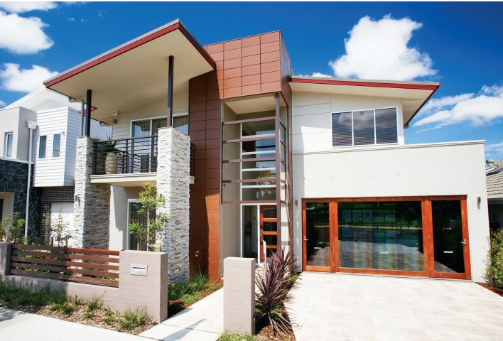
Contemporary homes at Rouse Hill demonstrate many of the principles outlined in these guidelines.
