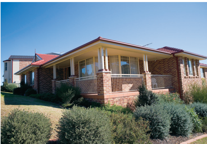
North facing verandahs can provide very enjoyable additional living spaces especially when they have a pleasant outlook.
