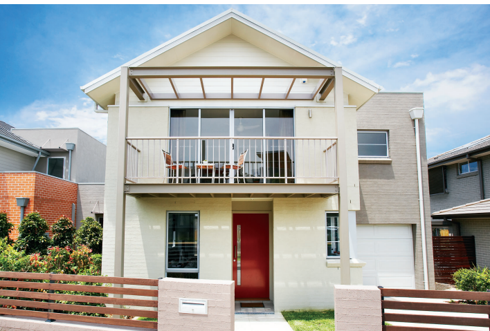
Providing a separate path from the footpath on the street to the front door is an important safety and amenity feature.
