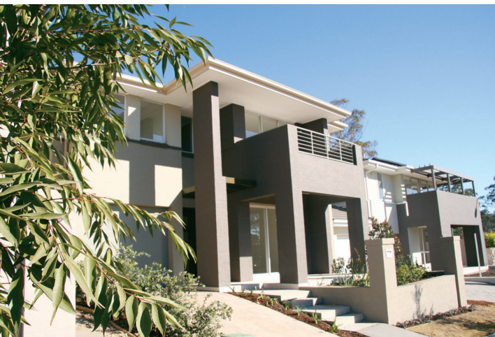
Layering and detail added to the front facade can add amenity as well as improving the appearance of the house from the street.
