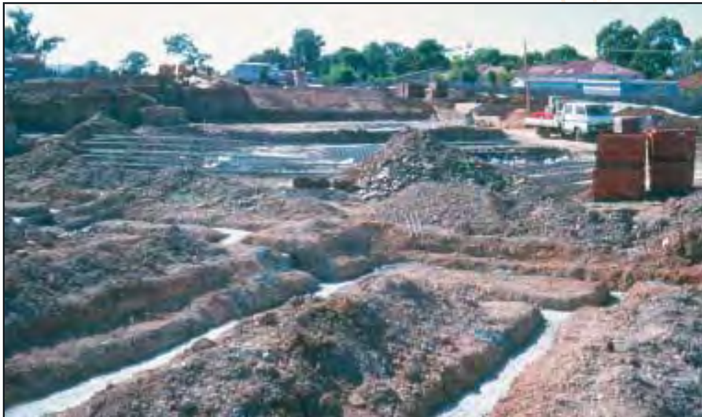
Figure 9.1 Typical medium-density, inner-city construction site.
