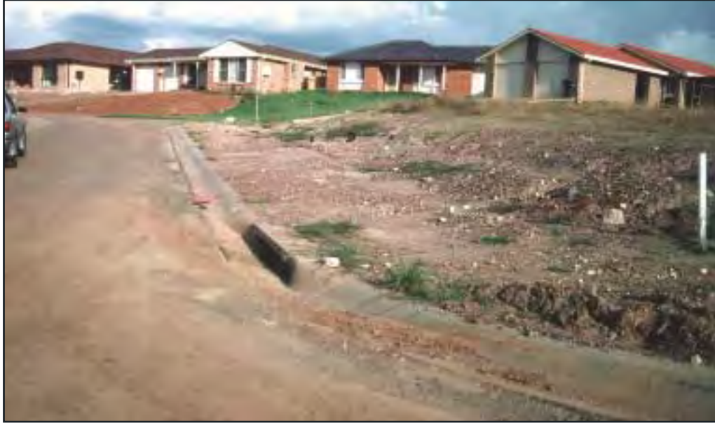
Figure 7.1 Unsatisfactory site stabilisation has resulted in substantial quantities of sediment leaving the site
