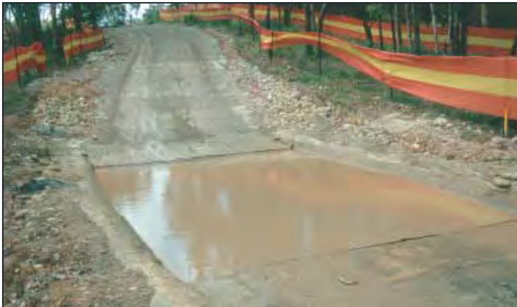
Figure 6.13 A simple wash-down system.
