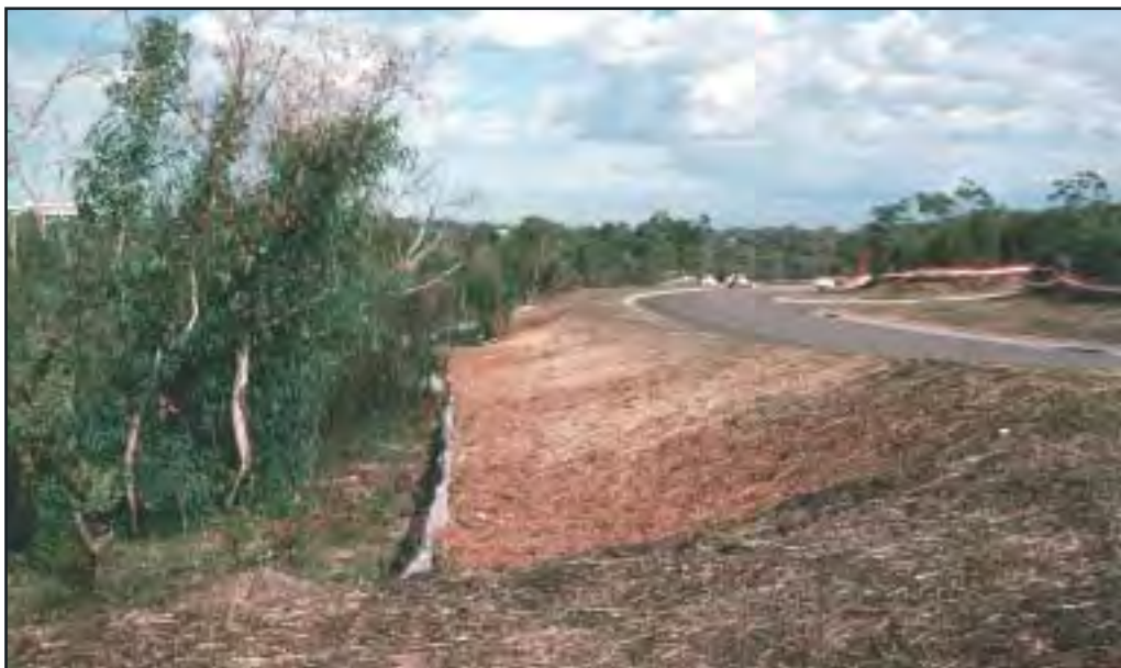
Figure 7.2 Primary revegetation of an earth batter with straw mulching (Section 7.4.1). Notice the sediment fence and barrier mesh to minimise soil erosion and sediment pollution
