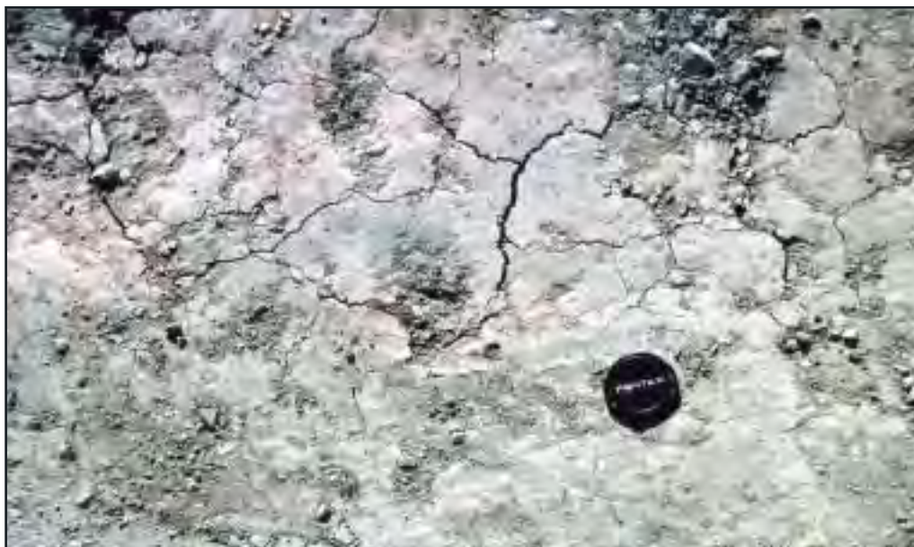
Figure A4 Smooth and compact ground surface typical of an urban construction site, raising the P-factor as high as 1.3
