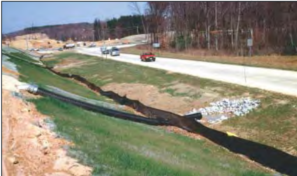
Figure 5.7 Use of heavy-duty flexible pipe to carry water down a batter
