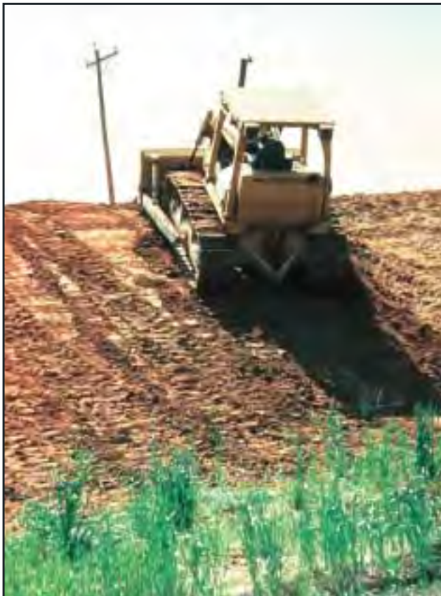
Figure 4.3(a) A track-walked slope (see footnote 4)
