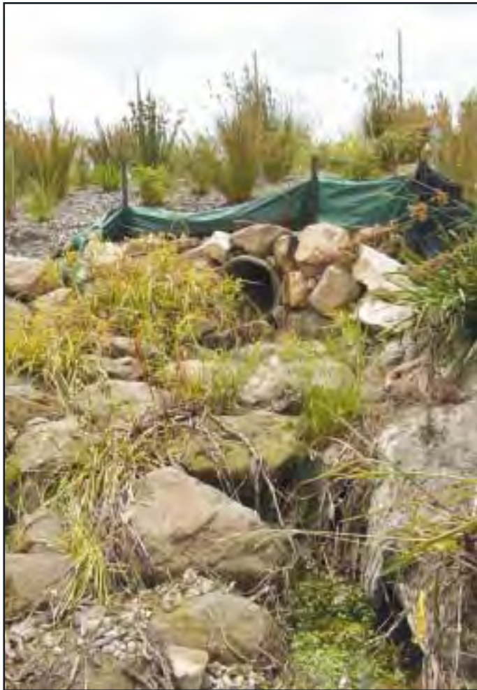
Figure 5.8 A riprap outlet on a steep slope.
