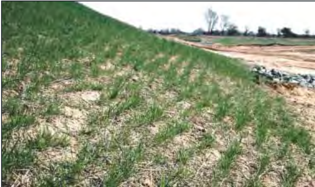
Figure 4.3(b) A track-walked slope (see footnote 4)
