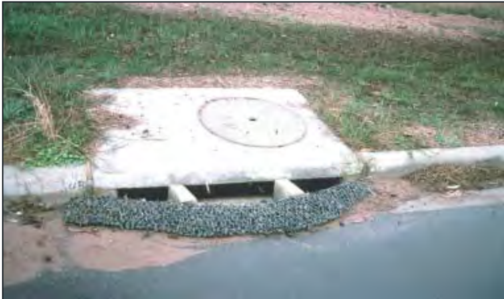
Figure 6.11 Filter roll at kerb-side sump
