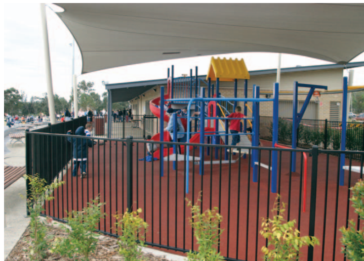
Where the safety of children, especially younger children may be at risk from the proximity of a playground to roads or where large crowds gather, fencing should be integrated into the design as seamlessly as possible. Photo - Hills Centenary Reserve, Sydney
