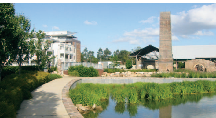
Reuse or redesign of existing waterbodies for water quality control and stormwater detention within new open spaces- as here in a former brickworks quarry – extends the community's association with the site's history. Photo – Holroyd Estate, Sydney
