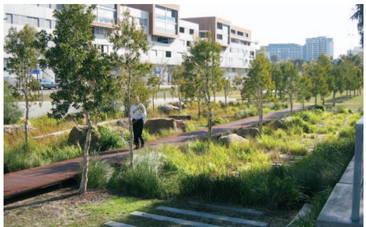
Vegetated swales: are constructed vegetated depressions that collect and direct stormwater runoff from impervious hard surfaces such as roadways, car parks and paving to areas that will benefit from irrigation. Photo – Vegetated swales, Victoria Park
