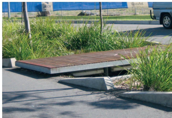
Water Sensitive Urban Design (WSUD) in practice at Victoria Park. Intermittent kerbing allows water to flow into vegetated swales assisting filtration of the urban water run-off. Strategically placed boardwalks maintain access through the space.
