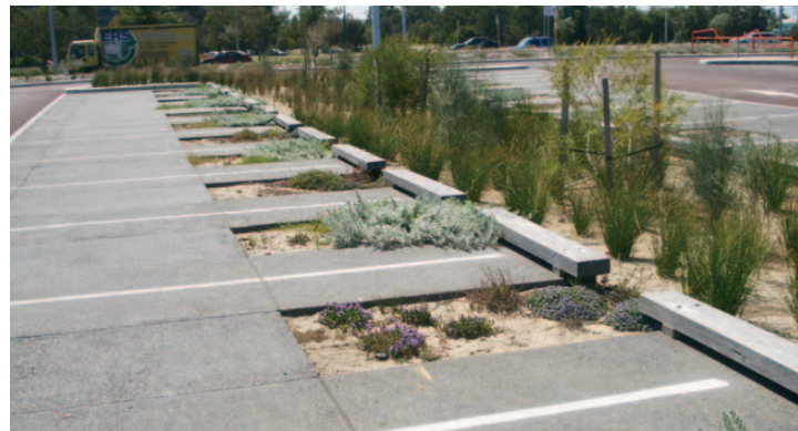
Maximising permeable surfaces reduces the volume of water entering creeks in storm periods. This can be particularly important in car park areas.
