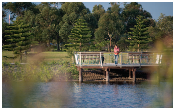
Simple built elements, such as handrails, ramps, sealed paths and tactile ground surface indicators can improve the accessibility of open space to people who have sensory or mobility disabilities. Photo - Koala Bay
