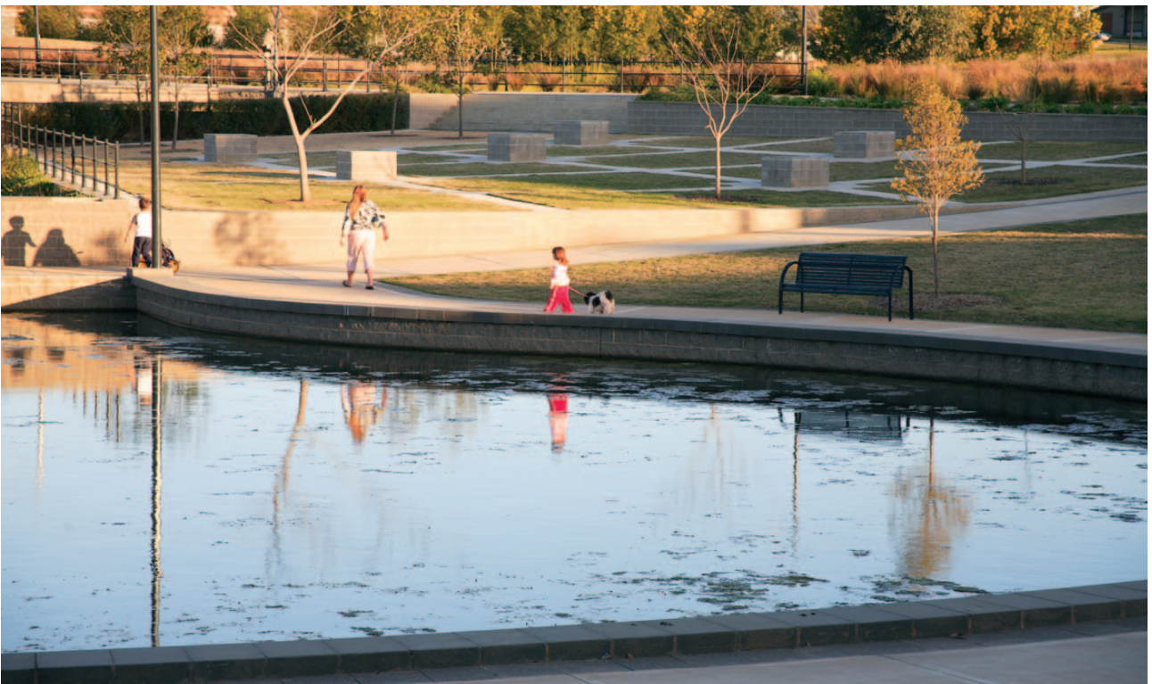
Feature water bodies that also have a hydraulic function in managing stormwater are common and popular elements in new residential developments. They bring with them numerous management issues that must be addressed with the End Owner from the outset. Photo - Park Central
