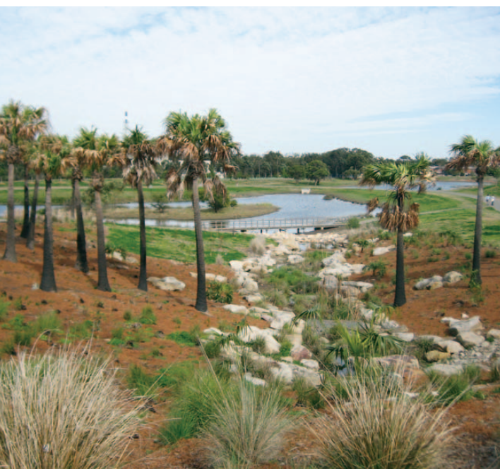
Where space permits, vegetated creek beds can perform an important water quality improvement role for receiving water bodies. Photo – Sydney Park
