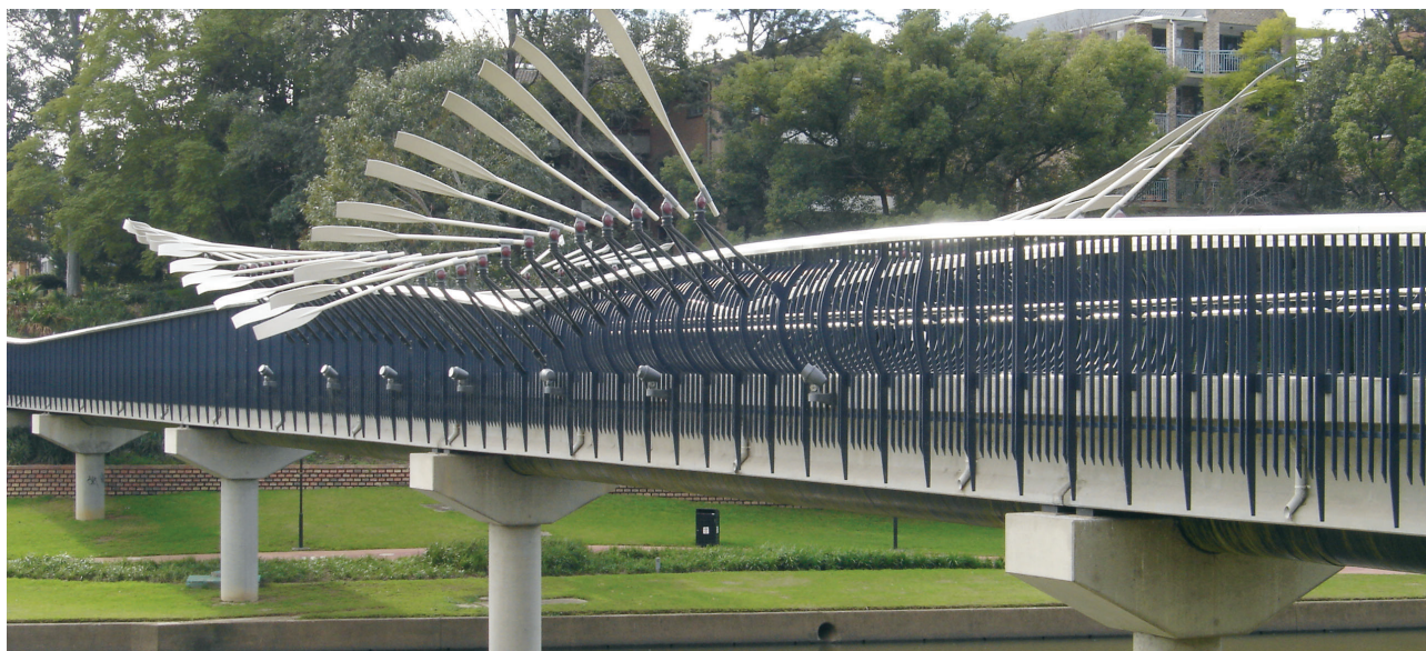
An elegant partnership between art and engineering, Milne Stonehouse's Bridge of Oars spans the Parramatta River providing pedestrian access to Parramatta's northern residential areas.
