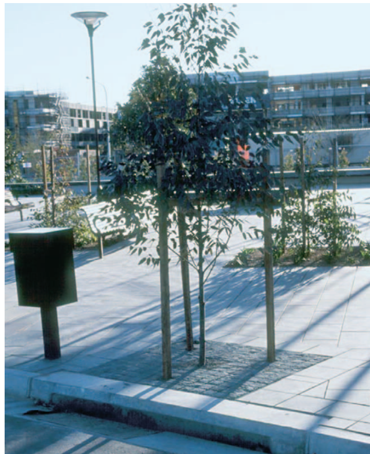
Here the upright kerb is part of a street tree bioretention system for trees in verges which can be a useful element within the WSUD strategy depending on the design, character and topography of the street.
