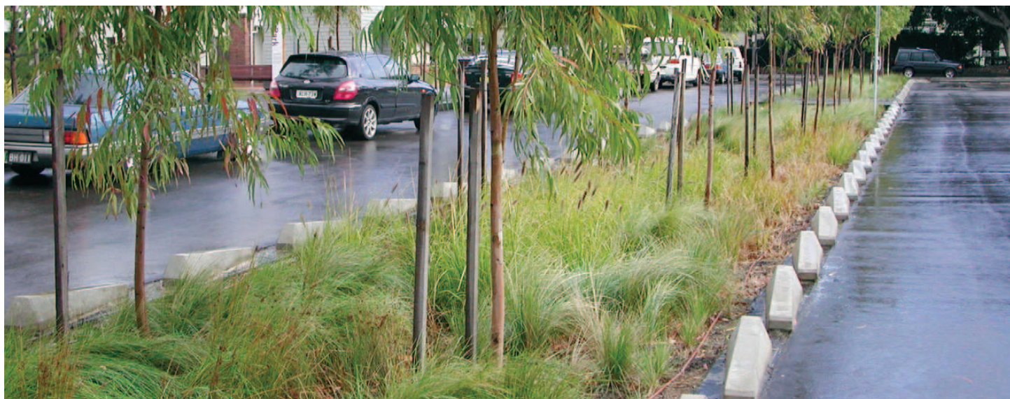
This street has a swale within its central median as part of the WSUD strategy. The unique kerb treatment and timber walkway also create an interesting streetscape.
