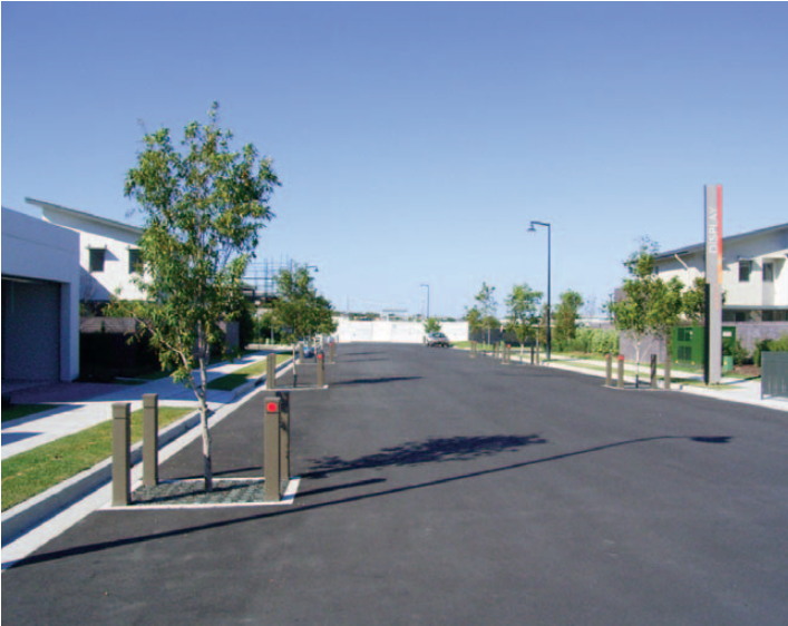
The tree guards in this street provide vertical elements that help to contain the street, until the trees are mature.
