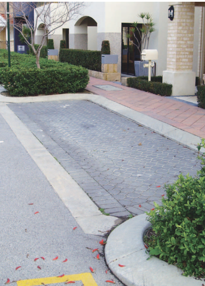
The parking bay is inset into the verge and separately defined from the carriageway.
