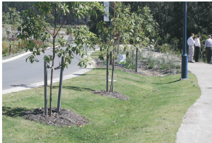
Swales can also be simple grass depressions on the street edge or within an open space area.
