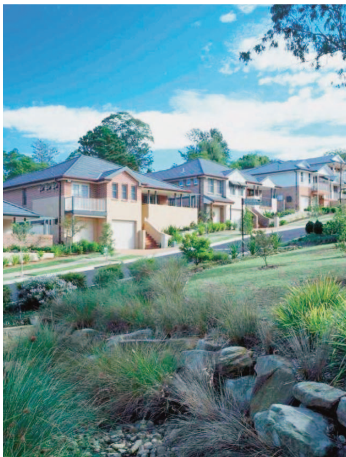
The dwellings in this street have absorbed the slope by being designed with the dwellings to have the garage on the low side of the block and the house wrapping over the garage.
