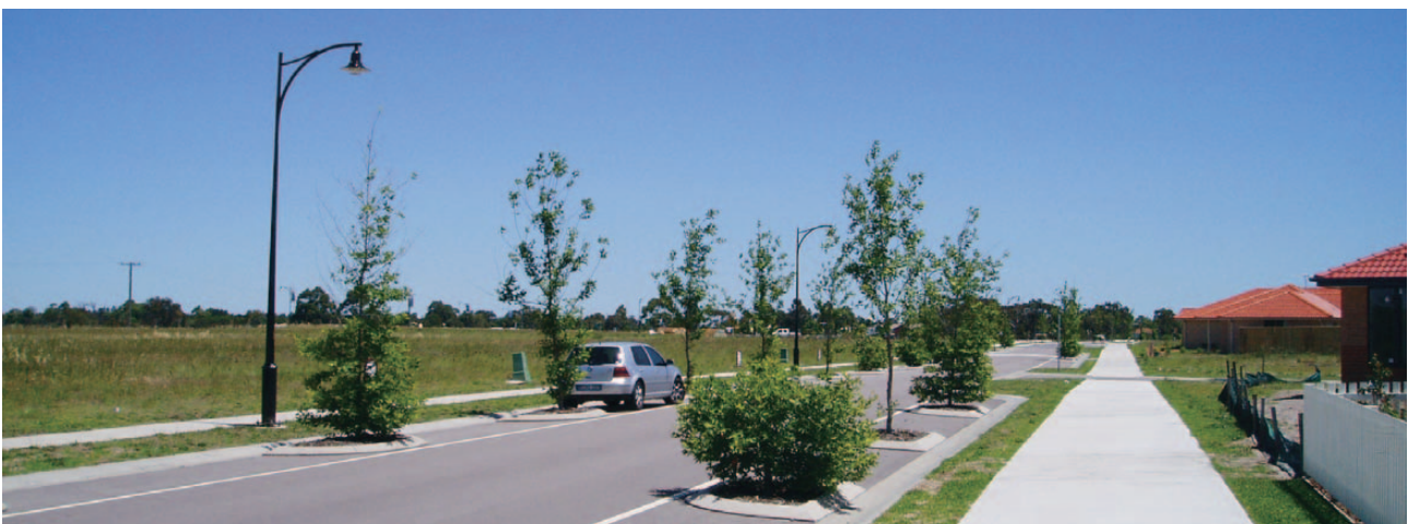
Although immature at present the trees between the car bays will provide a pleasant environment for this collector street. Here the cycle path has been combined with the footpath to provide a strong pedestrian link to the local centre.
