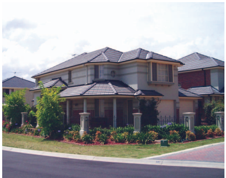
This house continues its front fence around the corner of the block with the higher rear fence set back along the building frontage.
