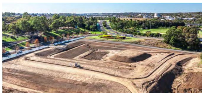
Macarthur Gardens North under construction
