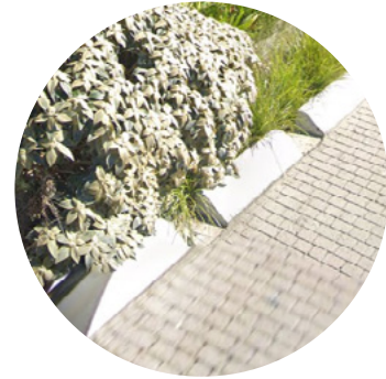
A swale with cut out kerbs
