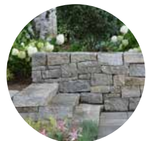
High Quality Retaining Wall
