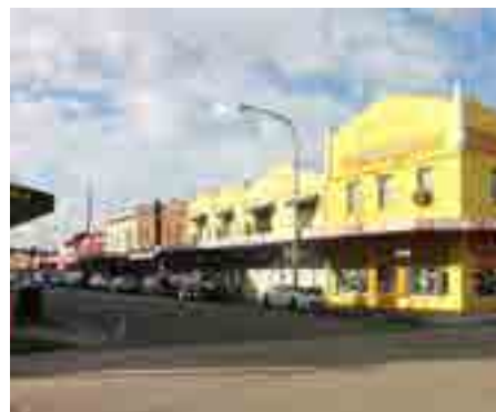
Figure 131. Existing local shops
