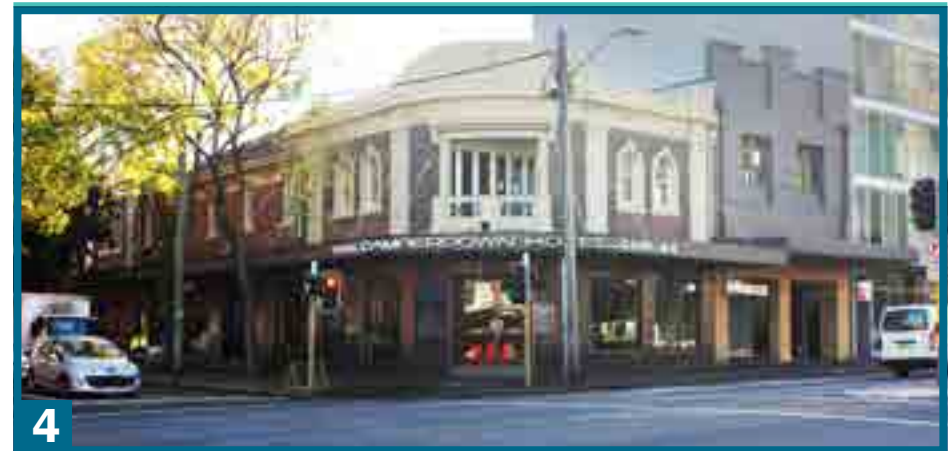
Figure 40. View of corner building on the corner of Layton Street
