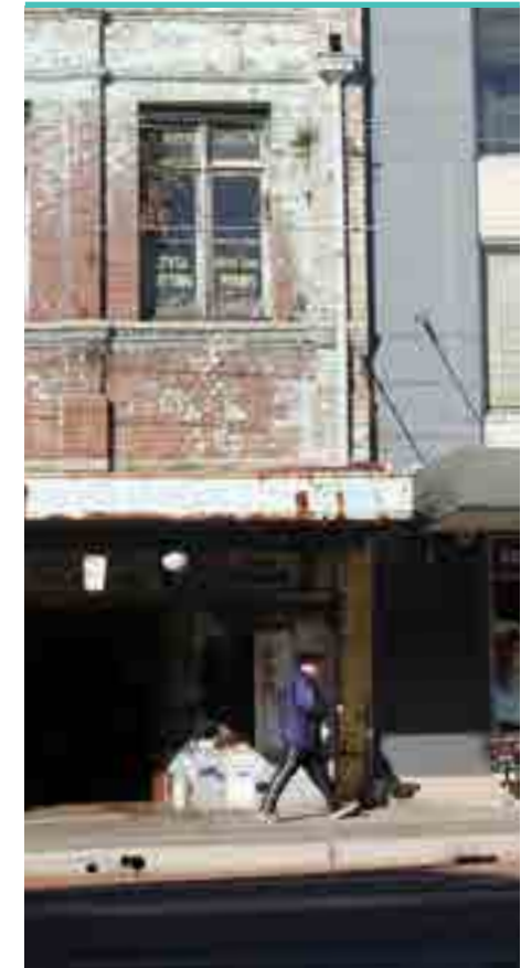
Figure 7. Facade detail, Parramatta Road
