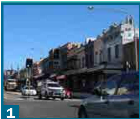
Figure 44. Shop top housing in Leichhardt
