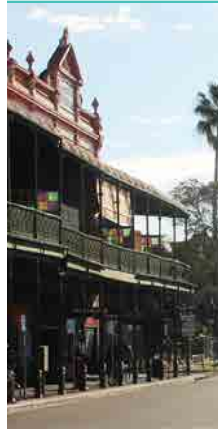
Figure 6. Facade detail, Johnston Street
