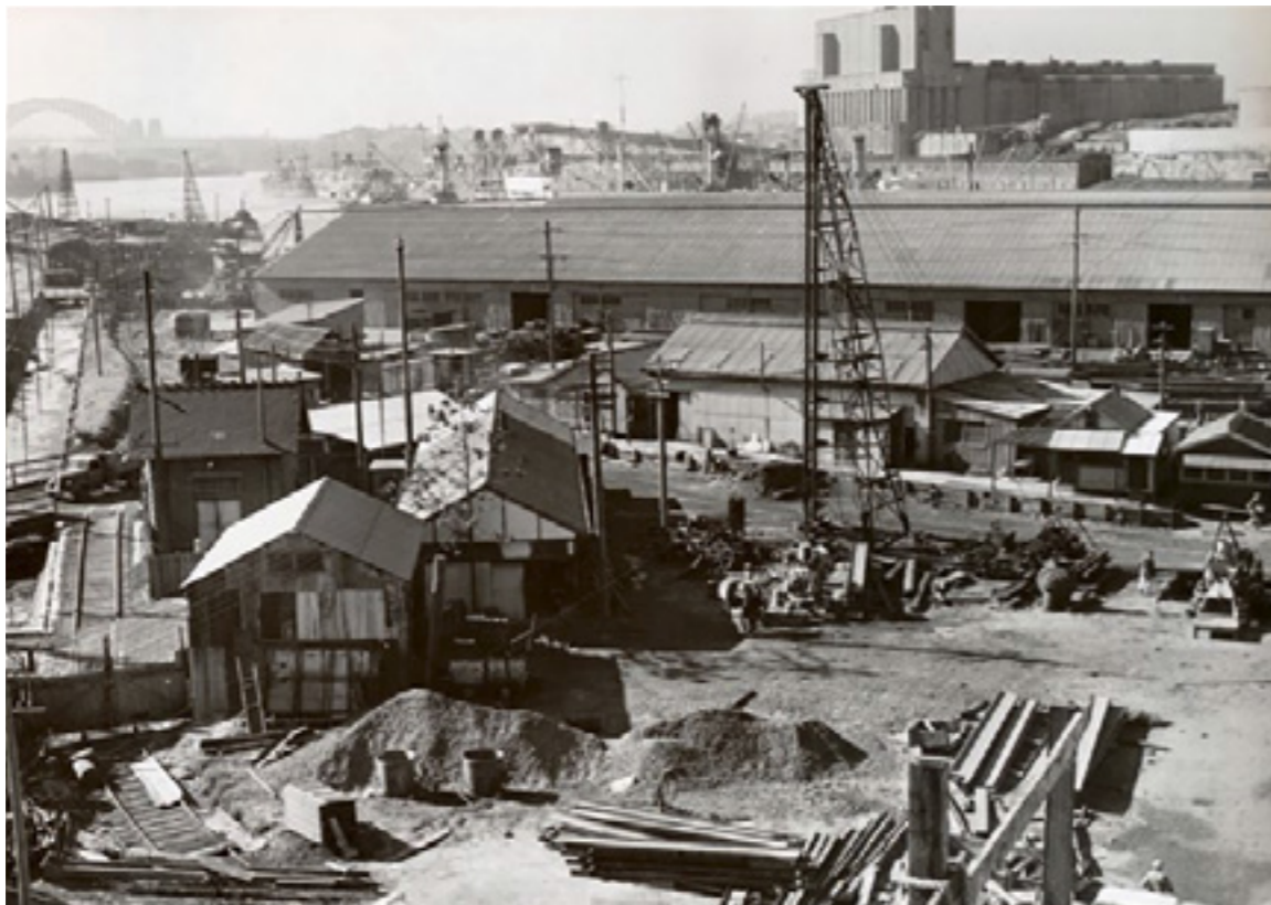
Material storage, WBPS.
