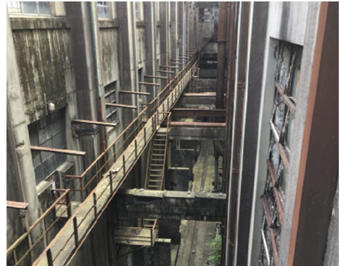
The catwalk between the boiler house and the workers club.
