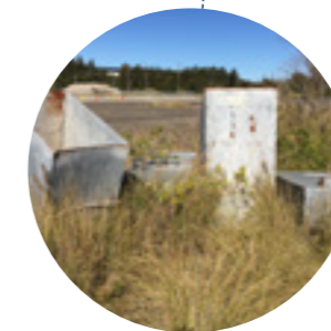
Steel ducting to remove
