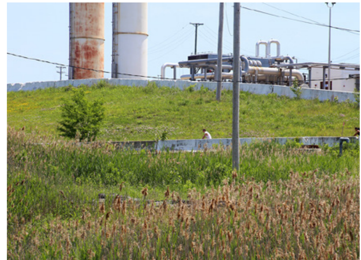
Image of the flare stacks in the background of a shared bike and pedestrian path. The stacks are not used, rather the captured methane gas is purified and used as an energy source. Image courtesy of Michael Anton. Taken from (Urban Omnibus, 2018).
