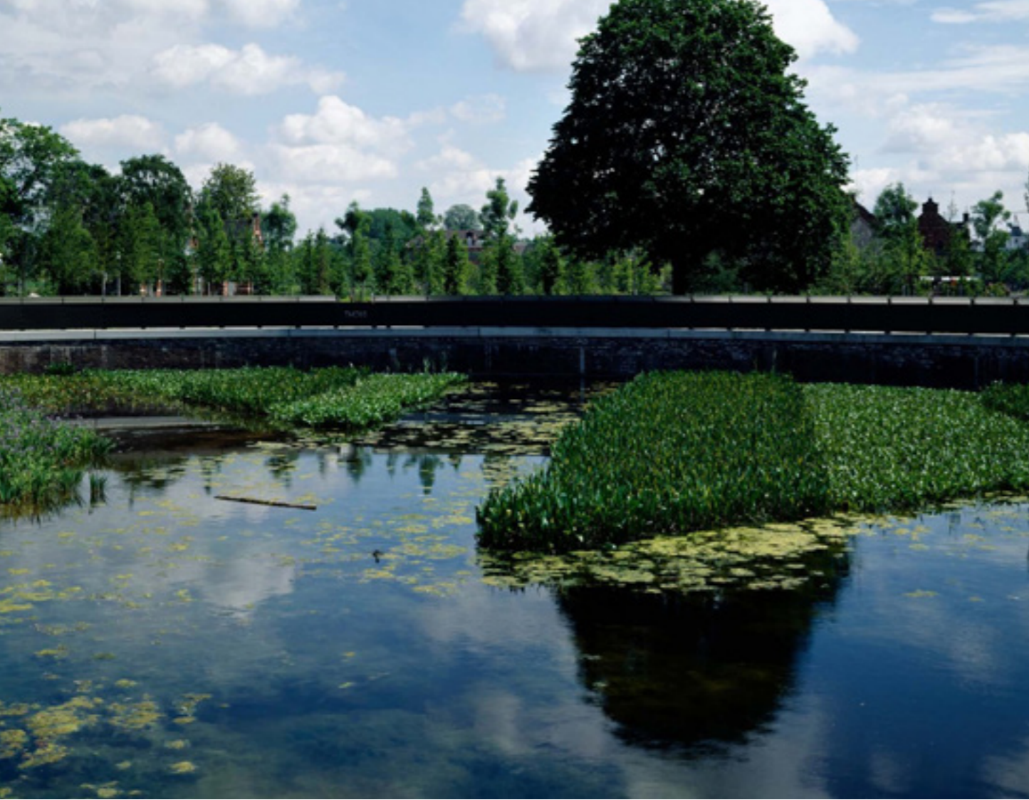
AFTER: Former Gas holder transformed into Aquatic and Water Lily Pools with floating timber walkways. Heavily polluted soil buried in foundations of Gasholder beneath concrete cap and aquatic gardens (Gustafson Porter + Bowman, 2006)
