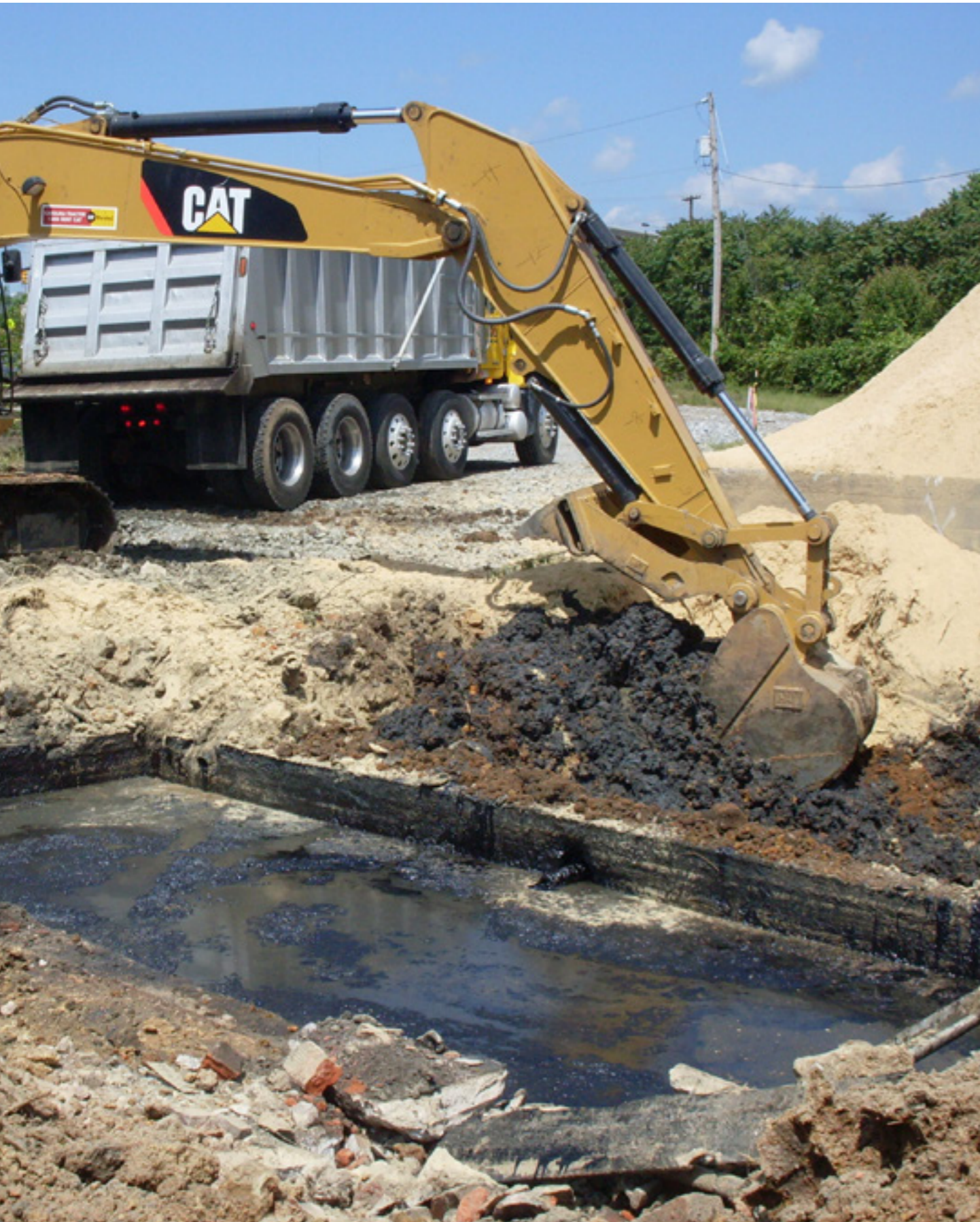
Example of soil contaminated with PAH's being extracted from a former manufactured gas plant in High Point NC. Image courtesy of NC DENR taken from ( https://sph.unc.edu/files/2014/10/High-point-orig-004.jpg )
