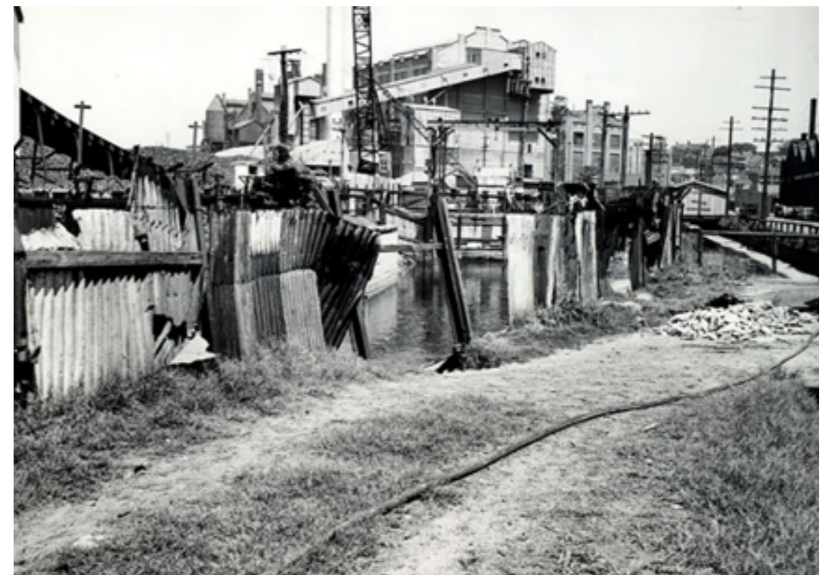
Cooling canal leading to the WBPS.
