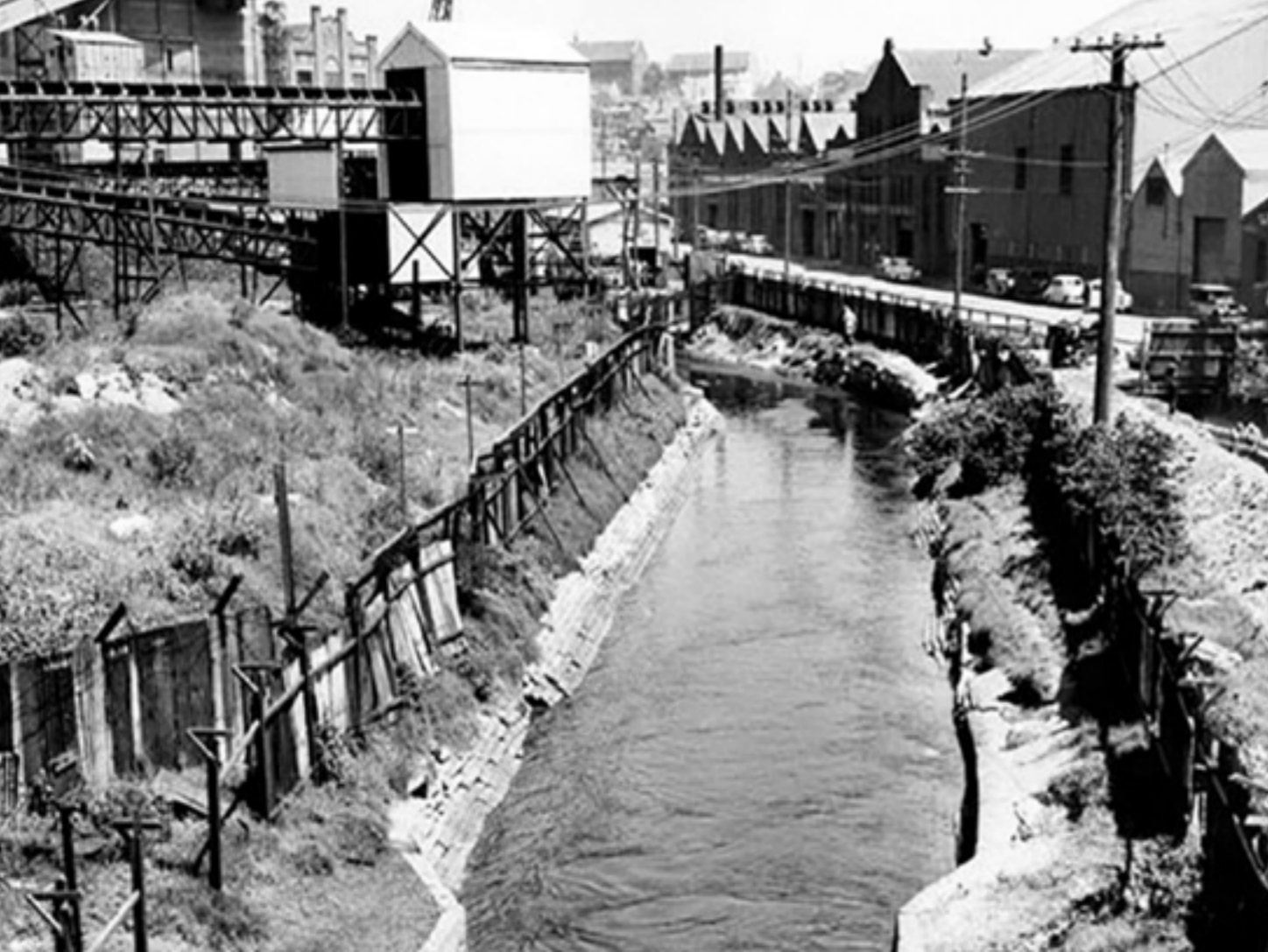
Cooling canal leading to the WBPS.
