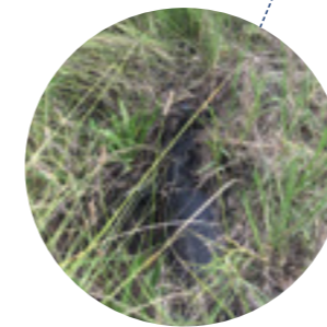
Large poly pipe to remove
